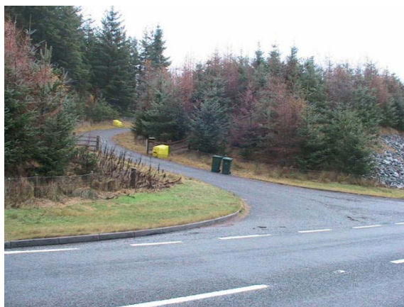
Fig. 4 : access to existing properties to the east of the A95
